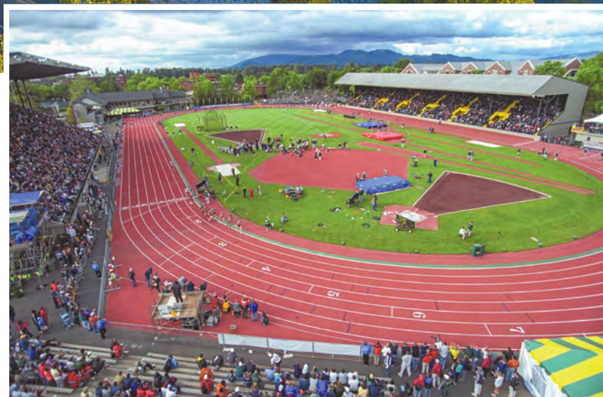
Before and after: The futuristic rebuild of legendary Hayward Field in Eugene, Ore., took three years and employed more than 250 members of Salem Local 280, whose handiwork was seen by millions of viewers in July during the World Athletic Championships.
